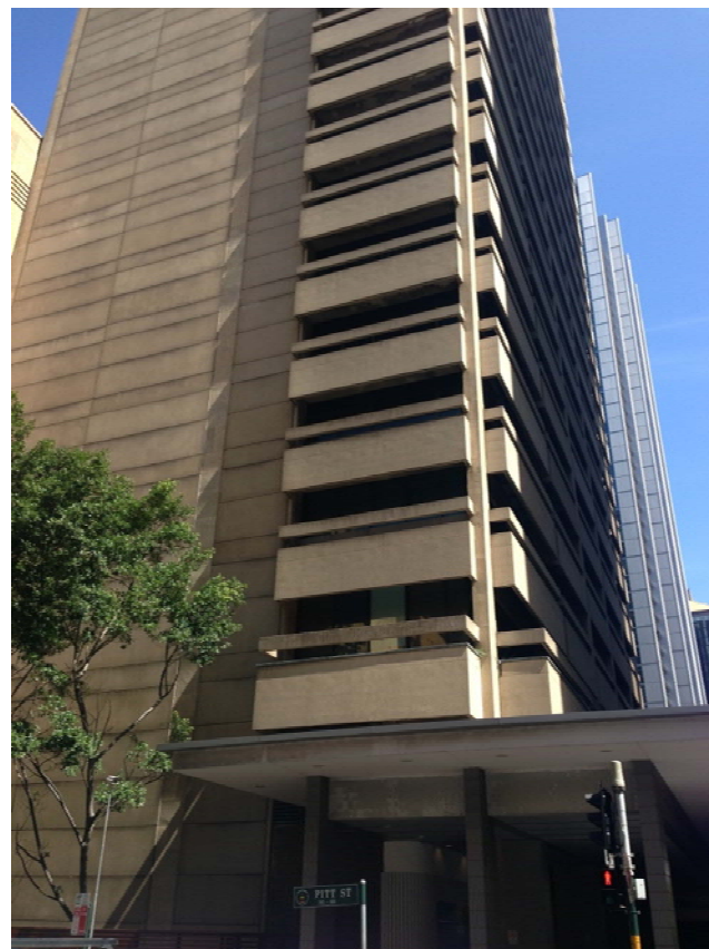
Figure 4: The eastern facade of the 1965 building
