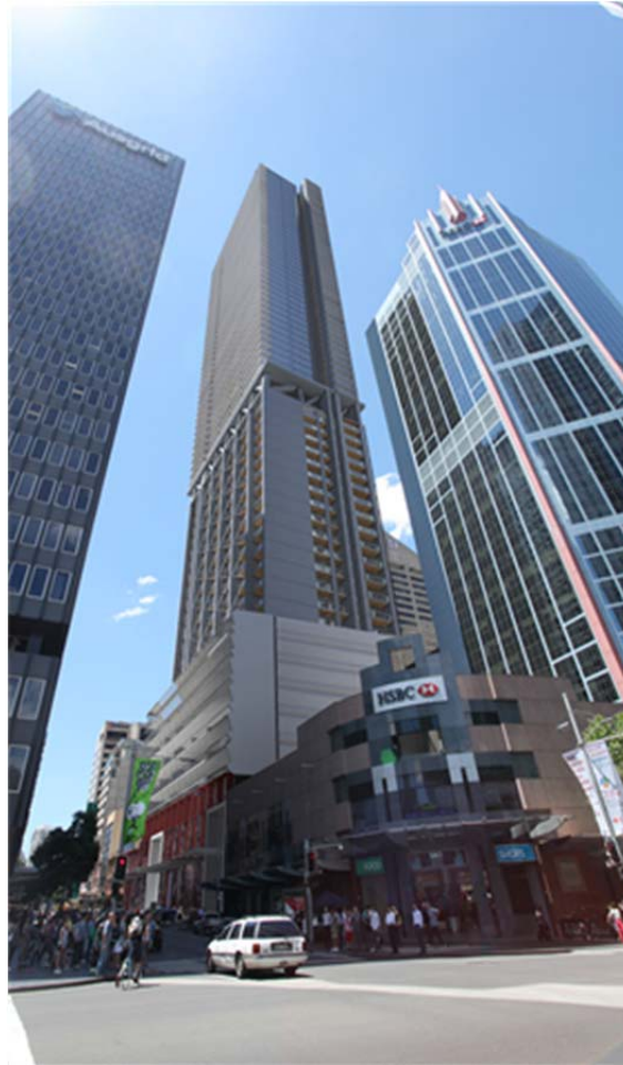
Figure 12: View from corner of George and Bathurst Streets
