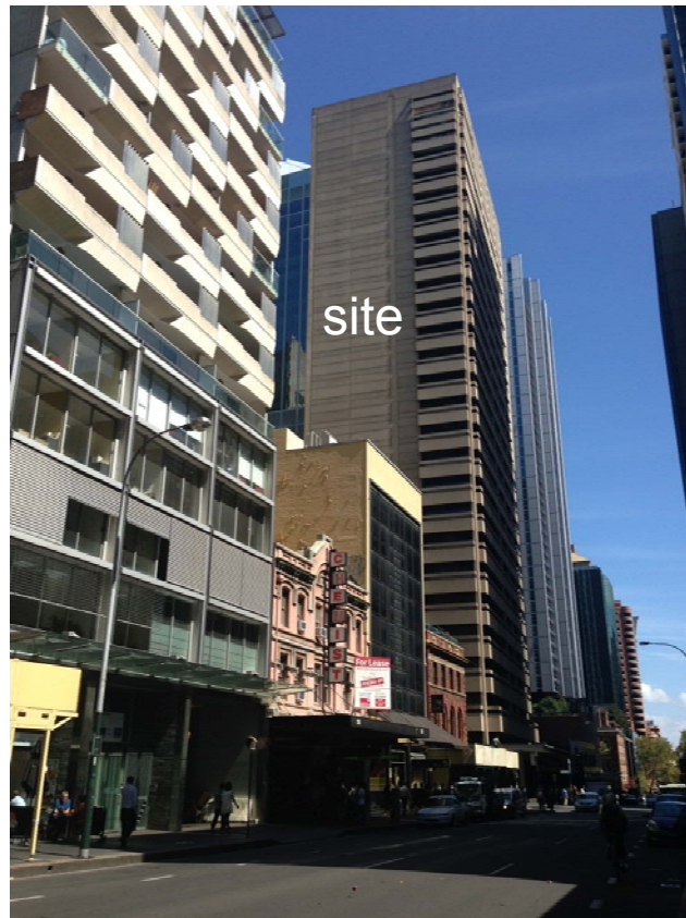
Figure 3: Looking west along Bathurst Street towards the subject site
