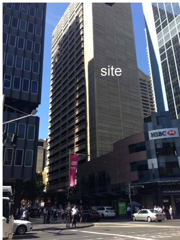
Figure 6: Site viewed from the corner of George and Bathurst Streets
